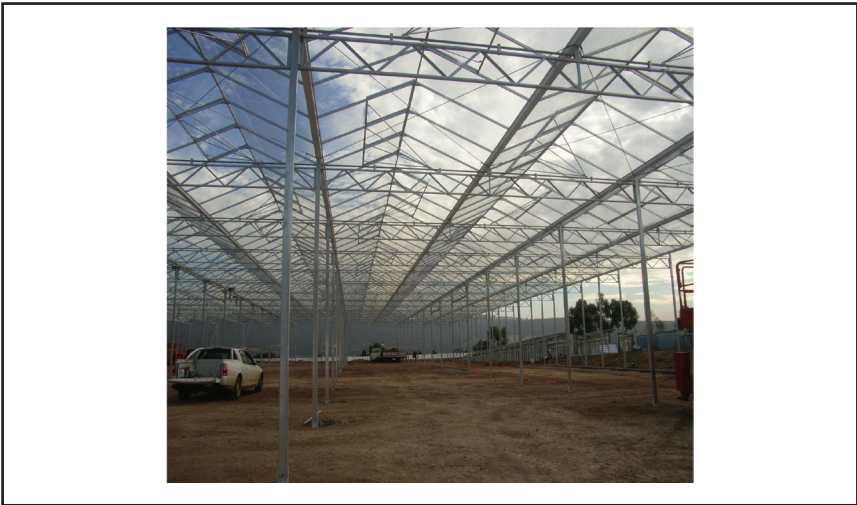
Figure 2. The new glasshouse under construction.
