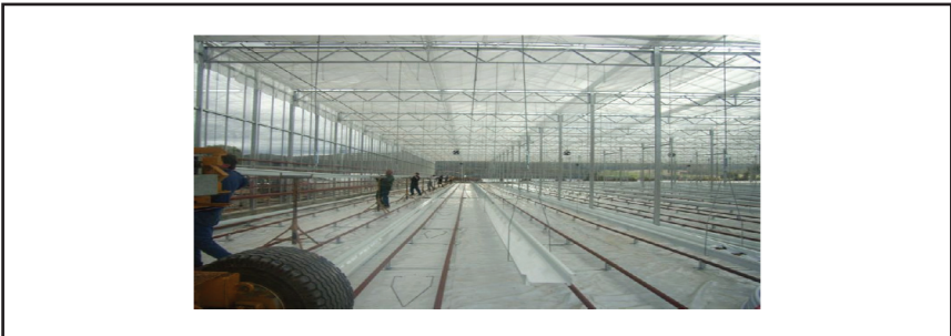
Figure 3. Internal equipment being installed.
