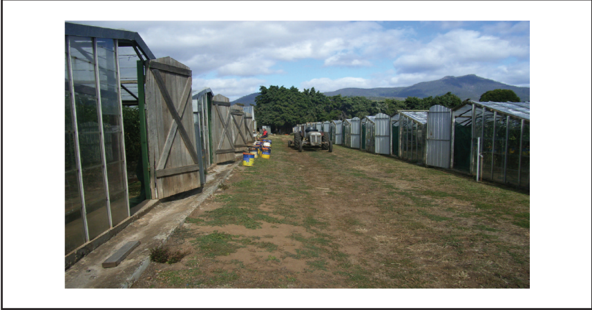
Figure 1. The conventional old wooden glasshouses before removal.
